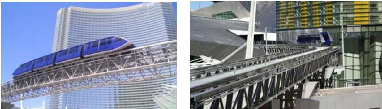
**Fig. 8:** DCC cable liner in Las Vegas and guide way with tubular joints
