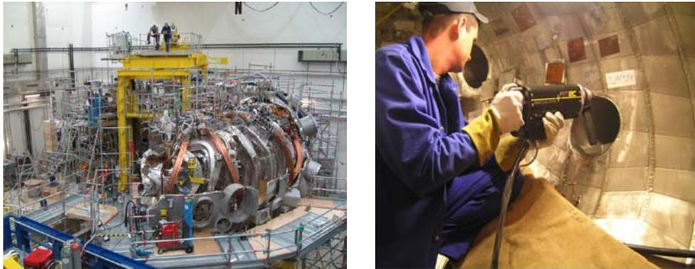
**Fig. 9:** Plasma vessel under construction and PIT treatment of each weld layer
